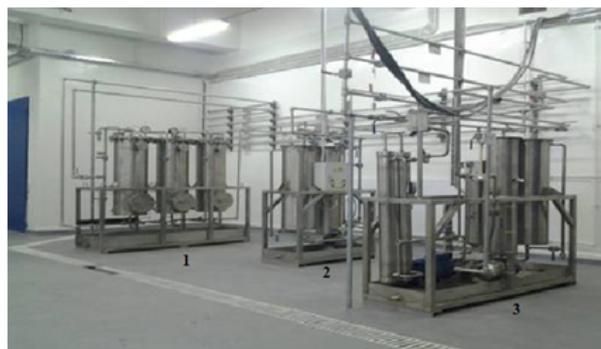
Fig. 1. AQUA-EXPRESS installation: (1) sand filtration module, (2) ultrafiltration module, (3) reverse osmosis module
