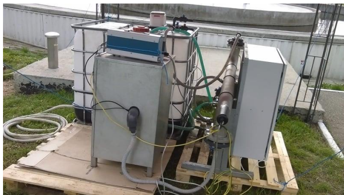
Fig. 1. Ultrasonic mobile pilot installation
